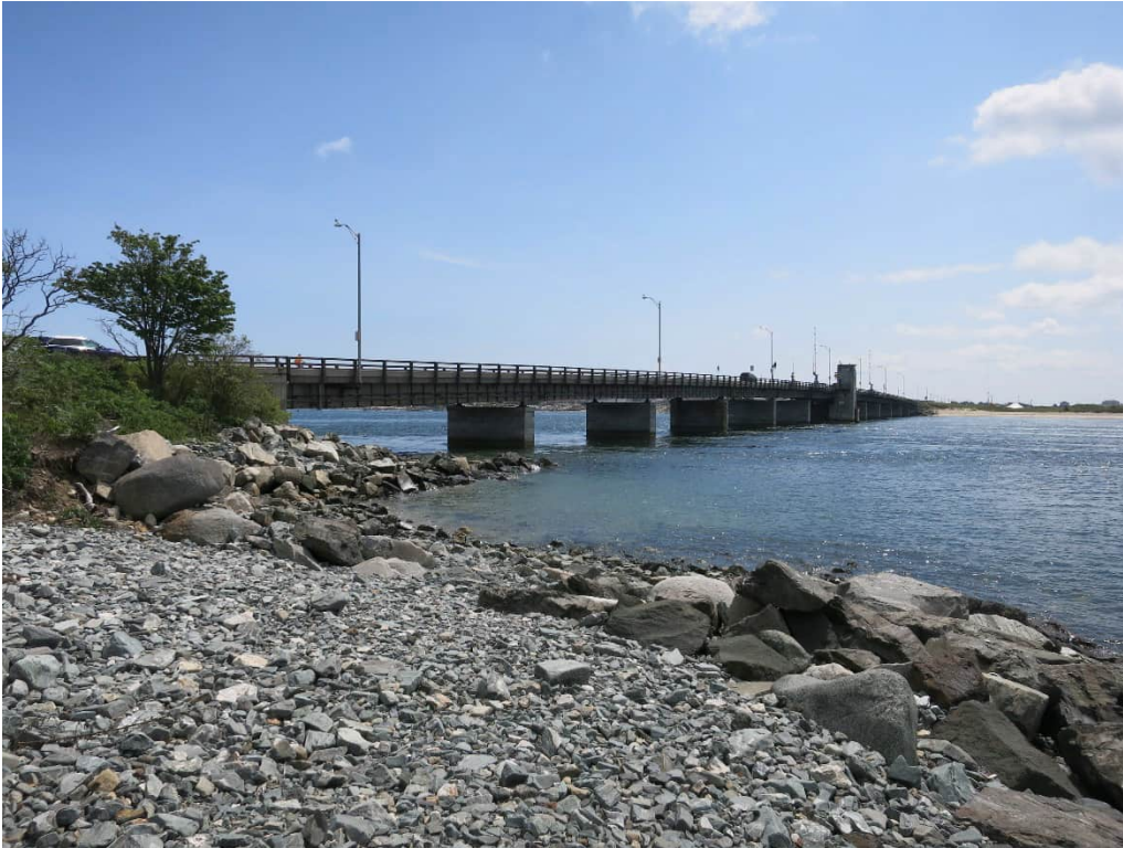
Photo 2. General view of bridge.
