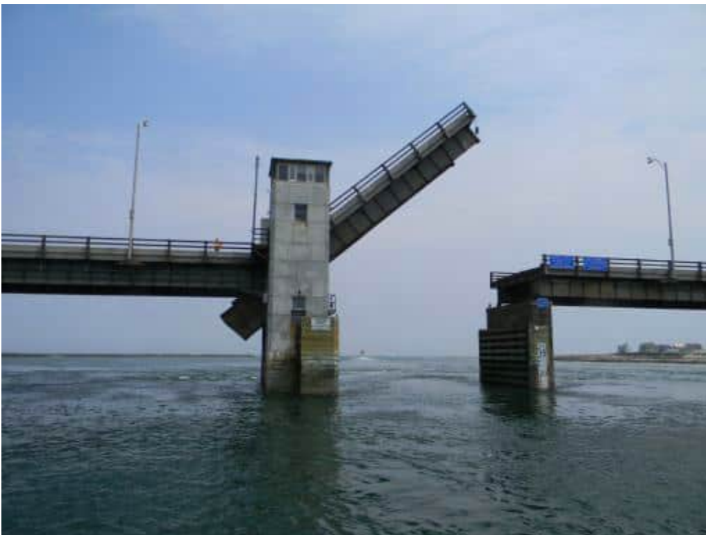
Figure 8. View of the bascule in the raised position (Bridgehunter.com).
