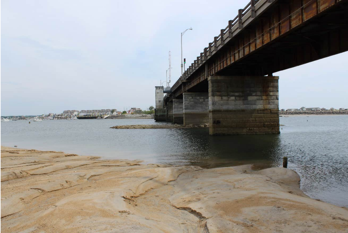
Photo 6. View showing low-tide exposure of bridge from south abutment.
