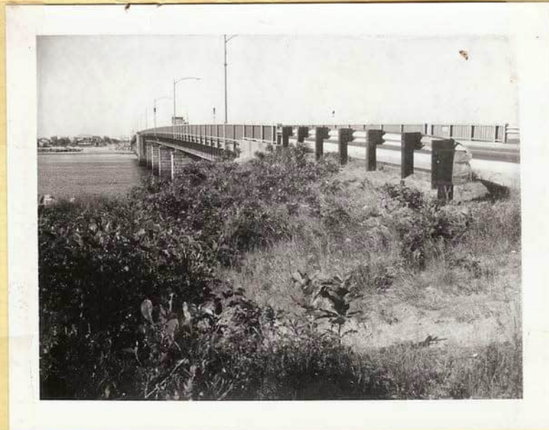
East Elevation Hampton End
