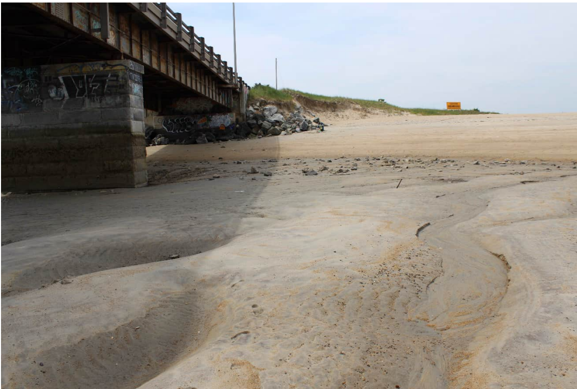
Photo 5. View showing south abutment and one of the piers.
