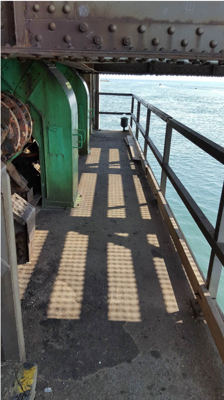
Photo 9. Catwalk under movable deck.
