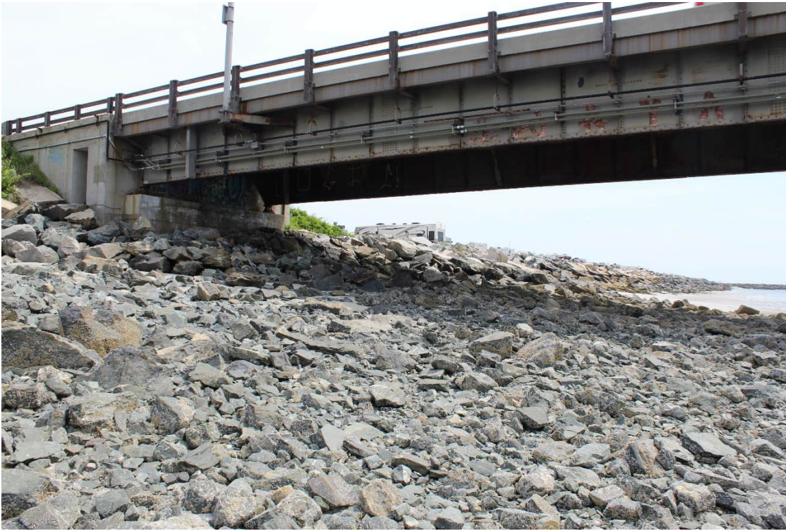
Photo 4. View showing north abutment and underside of superstructure.
