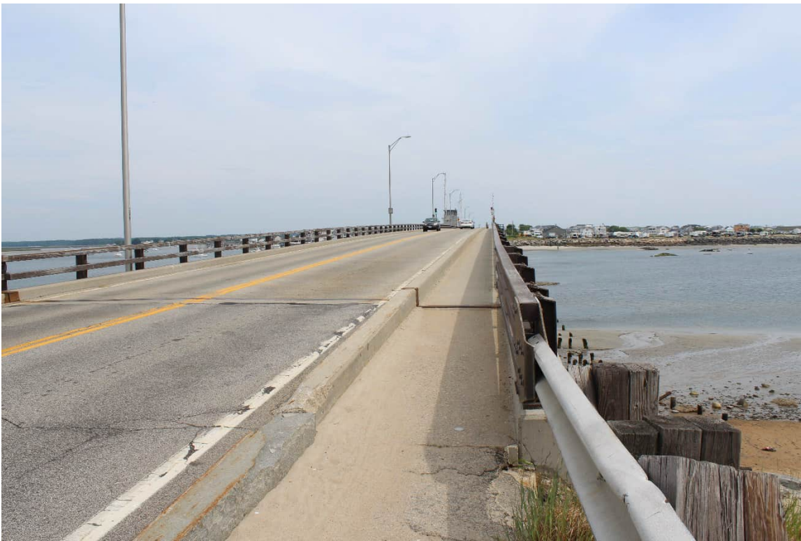
Photo 7. Deck from south approach.
