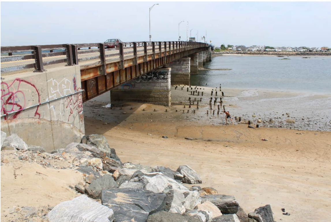
Photo 11. Southeast quadrant of the Neil R. Underwood Memorial Bridge. Note wooden pilings visible at low tide, extending north from Pier 6-S.
